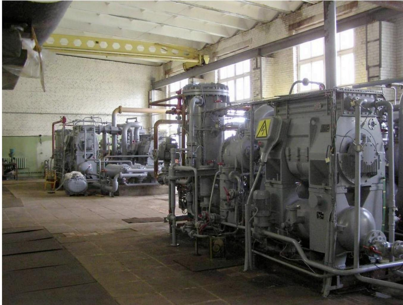
**Additional screw compressor for helium (6000m<sup>3</sup>/h) - from HELIIMASH
